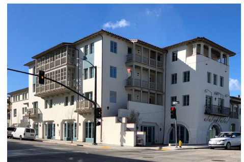
FIG. III.B.2: CONCAVE CORNER This concave corner creates space for a small retail court at the ground floor.
