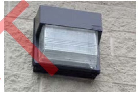
FIG. II.F.2: PROHIBITED LIGHTING Wall Pack lights on building facades are prohibited.
