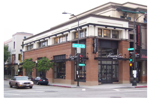
FIG. III.C.1: UPPER-STORY STEPBACKS The fourth story of this building steps back to respect the prevailing height of existing buildings on this street.
